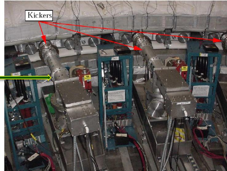
These are being replaced to have a "kick" over a smaller time period to produce a more stable beam.
