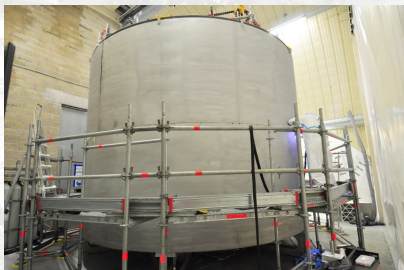
Jul/Sep 2013: IV vessel, IV PMTs, buffer vessel welding and installation into IV
