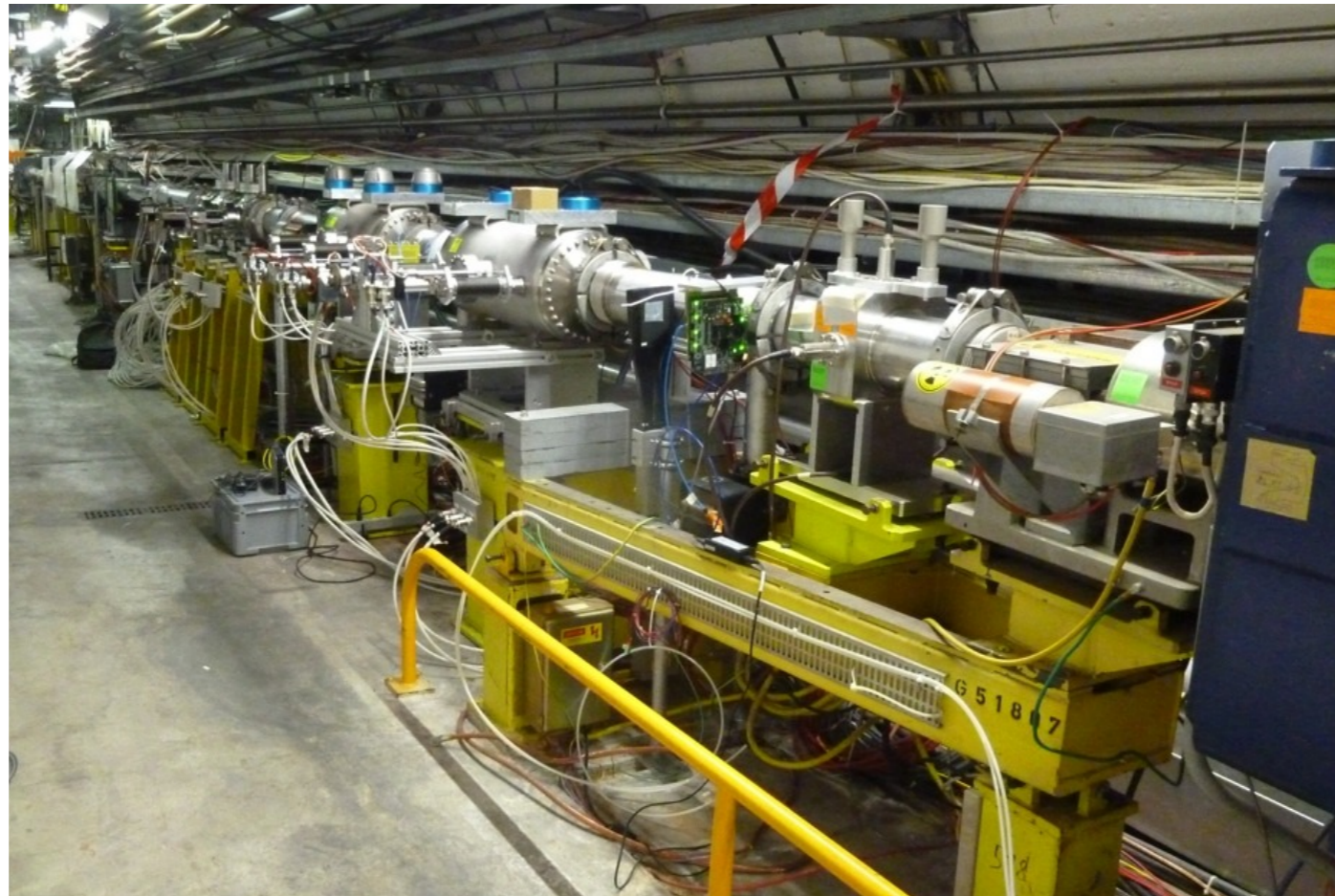
UA9 installation in the SPS
