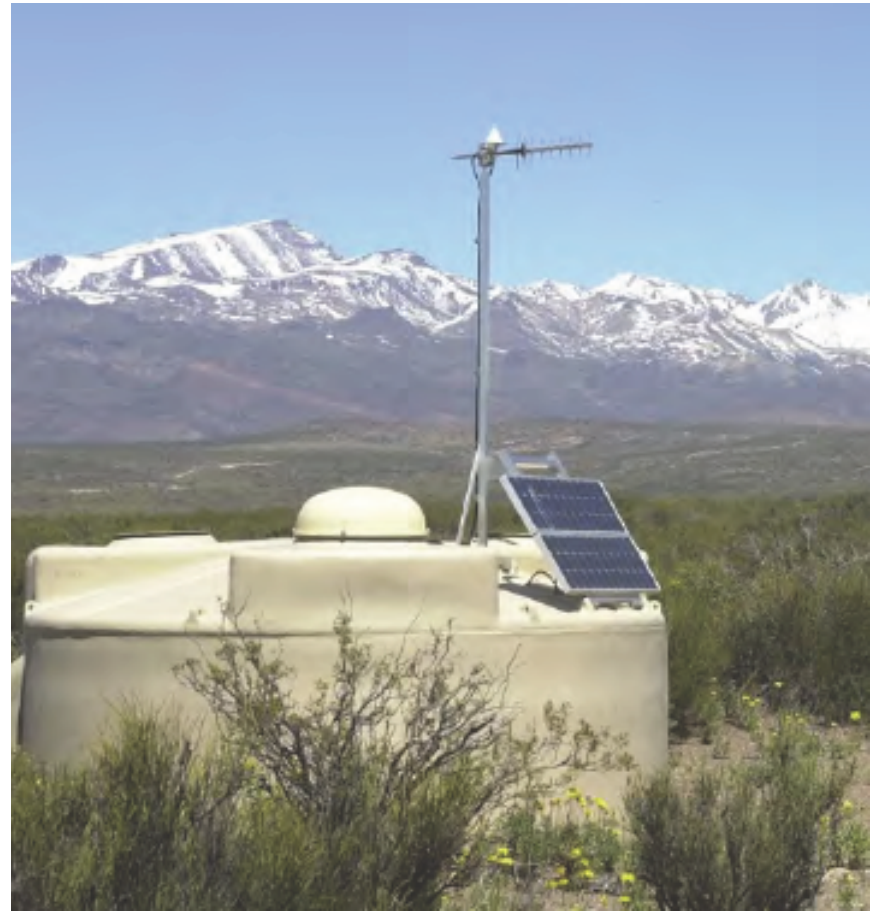
3.6 m diameter water tank containing a sealed liner with a reflective inner surface. 12 000 l of ultra-high purity water. Three 9 inch PMTs, Photonis XP 1805, look downwards through windows of clear polyethylene.
