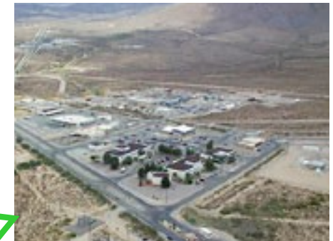
White Sands Ground Terminal, NM
