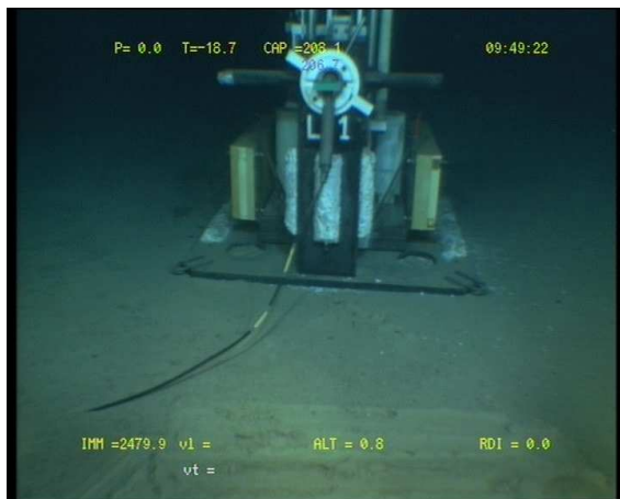
Fig. 2. An interconnected string anchor
