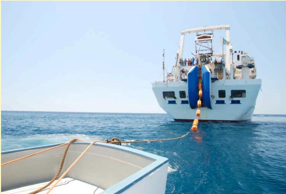
*Laying of the Main Electro-optical cable's shore-end at Portopalo*
