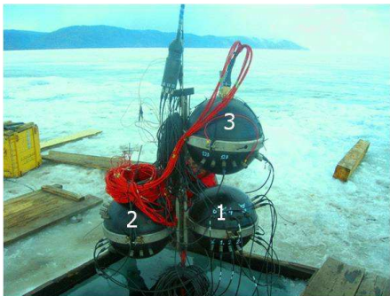
Fig. 10. FADC sphere (1), String PC unit (2), and LED flasher sphere (3) after final installation
