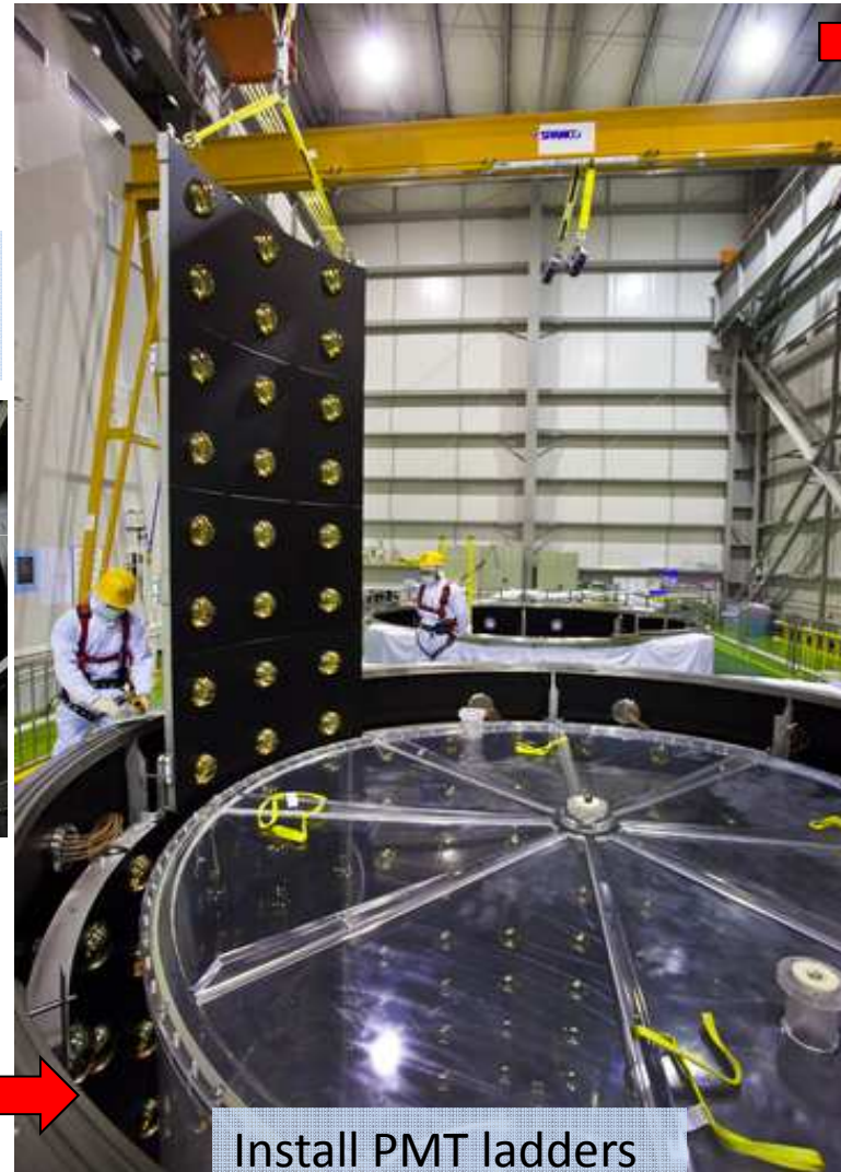
Install lower reflector
