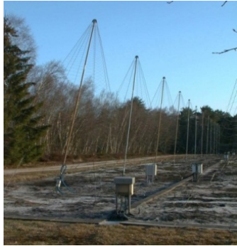
Log-Spiral Antenna (2005) Circular polarization Diameter = 5m Heigh = 6m
