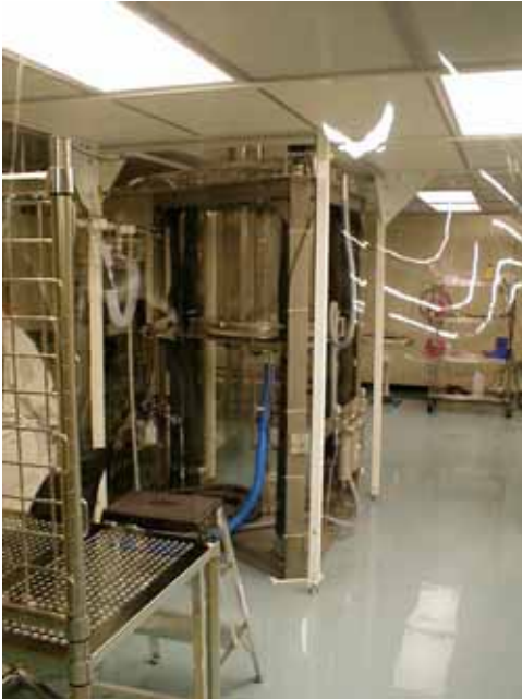
Spray-wash system for RF cavities (@FNAL)
