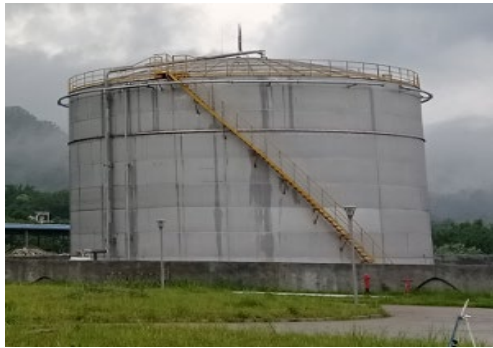
5000 m 3 LAB storage tank
