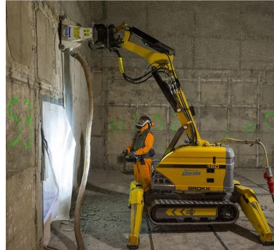
Remote-controlled demolition robot — EWN GmbH
