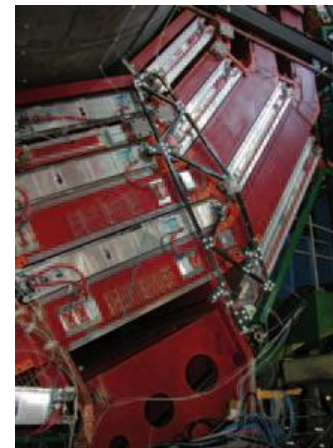
Installation des structures
