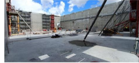
View of the DESIR construction site by mid-May 2024
