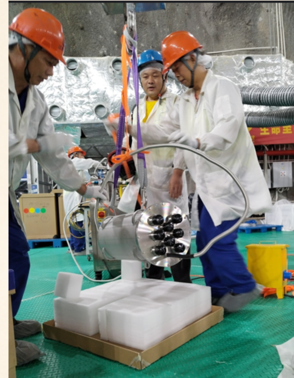
Underwater box lifting and installation
