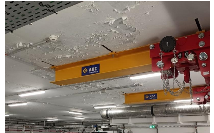
Roof of the HRS room
