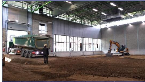
Construction started early 2020
