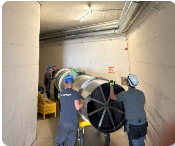
Handling & transport of 6 m sections into TT4
