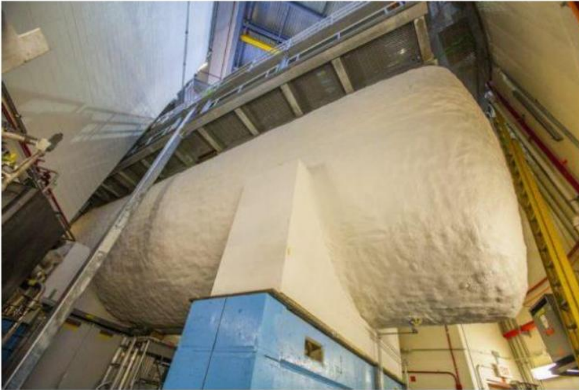
Cylindrical cryostat on support system covered in insulating foam during operation.
