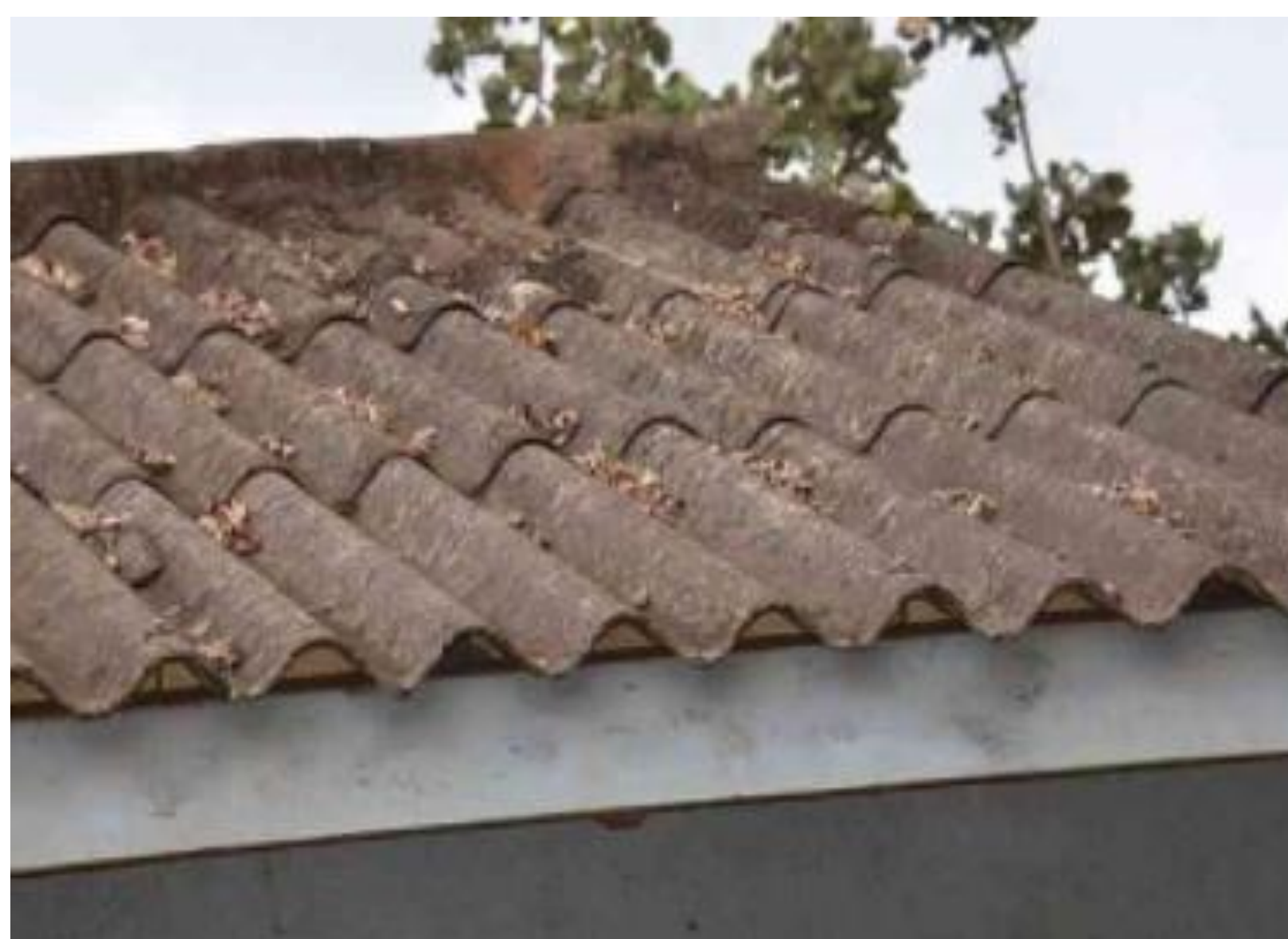
Fig. 2 Asbestos roofing
