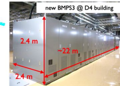
New Power Supply for MR main magnets
