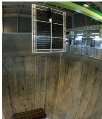
TOF installation (July 2023)
