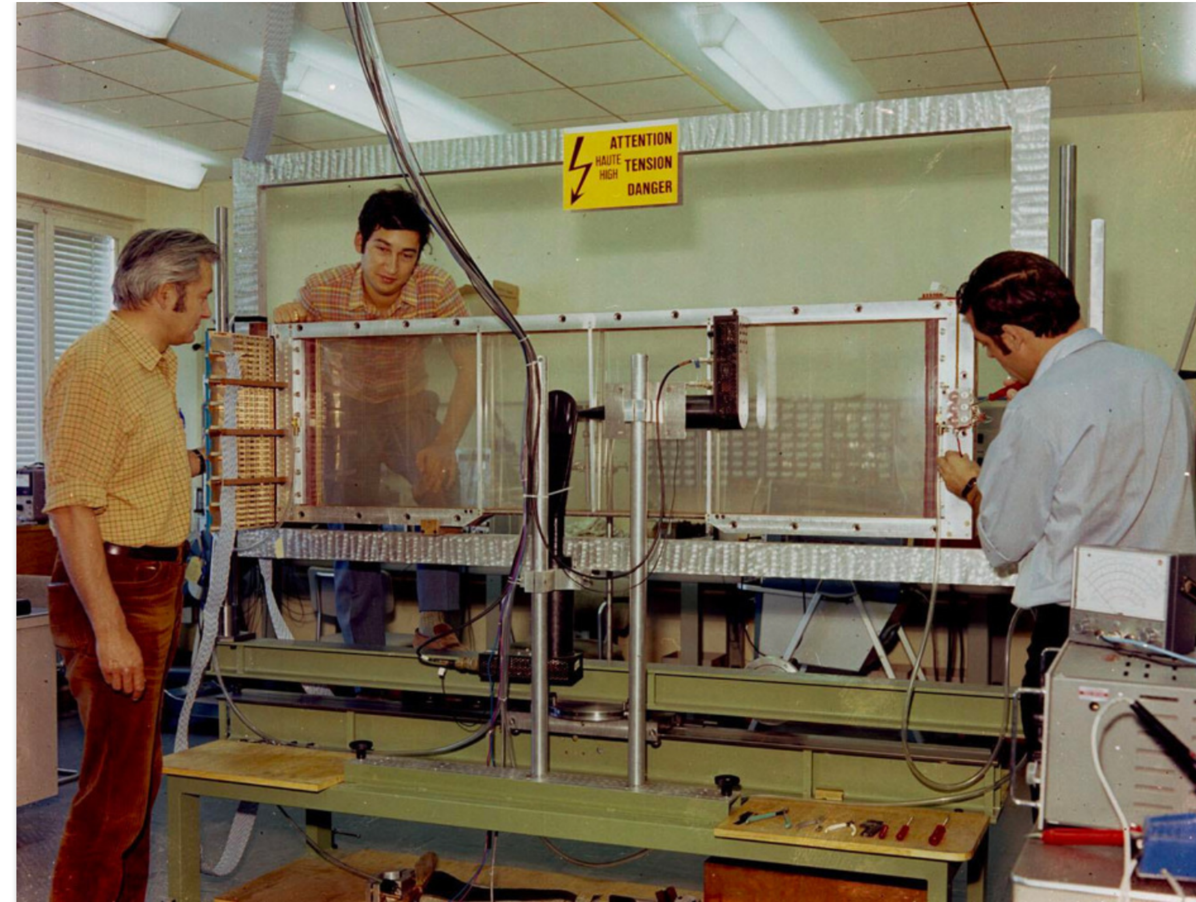
Georges Charpak's 'multiwire proportional chamber' particle detector consisted of many parallel wires, each connected to individual amplifiers. Linked to a computer, it could achieve a counting rate a thousand times better than before (Image: CERN)
