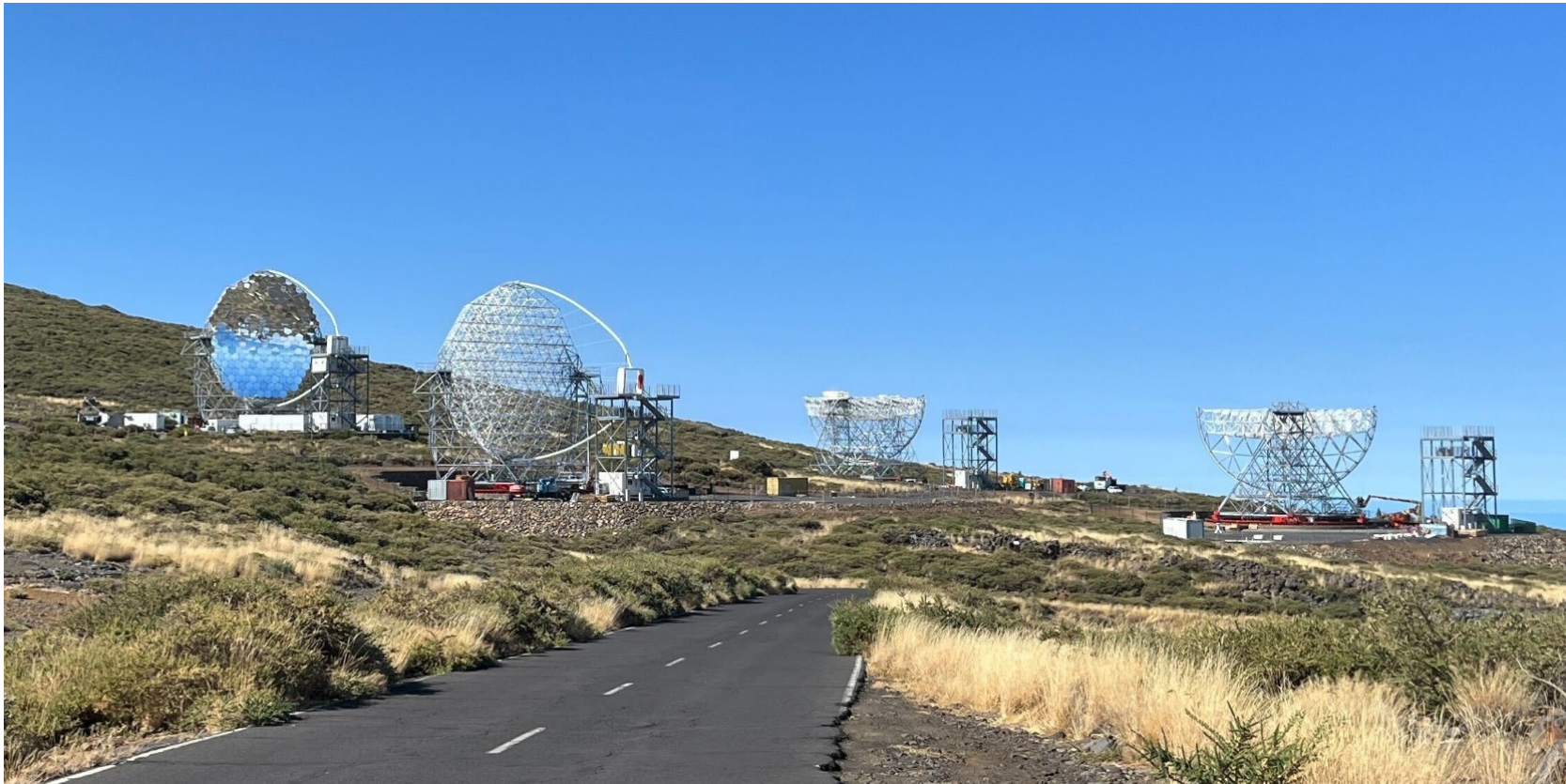
Picture of the CTAO North site, with the 4 LSTs (September 2024)
