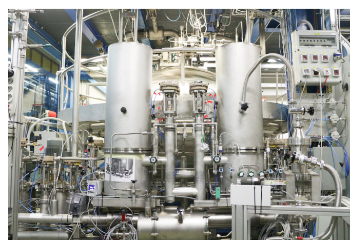
Liquid xenon purification system
