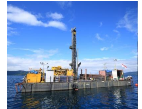
Drilling works on the lake
