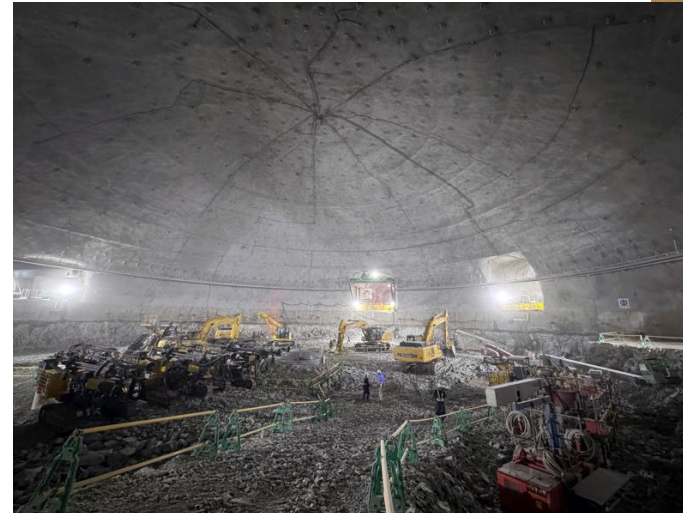
Progress of the excavation (end 2023)
