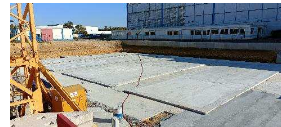
October 2023 : surface preparation
