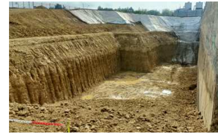
July 2023 : general earthworks
