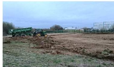
April 2023 : surface levelling
