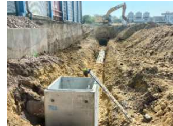
June 2023 : reorganization of site utilities
