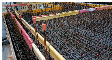
October 2023 : steel reinforcement level -3
