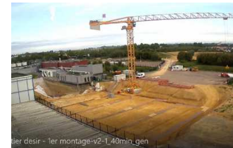
September 2023 : site preparation
