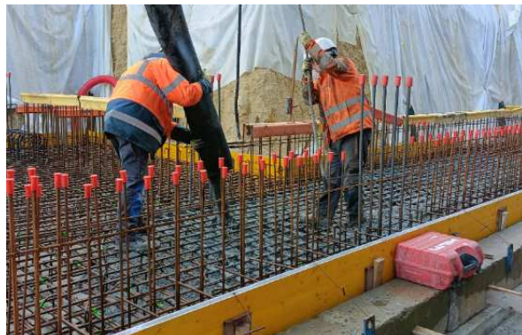
31 October 2023 : first concrete!
