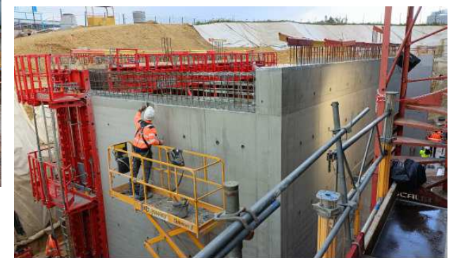
January 2024: Finishing of level -3 wall
