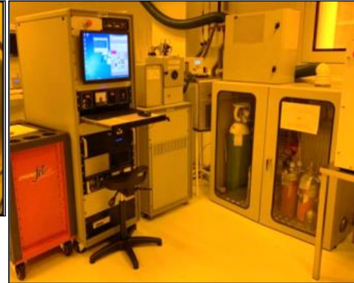
RIE machine on the Nanofab platform (PLASSYS)
