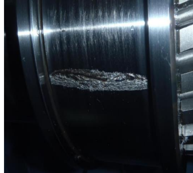
A damaged bearing on the main shaft of a wind turbine – Courtesy of Engie Green
