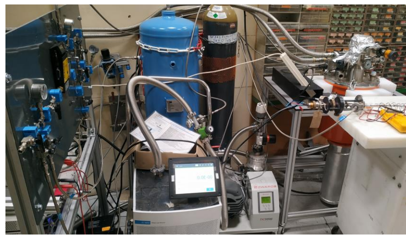
Other cryogenic equipment
