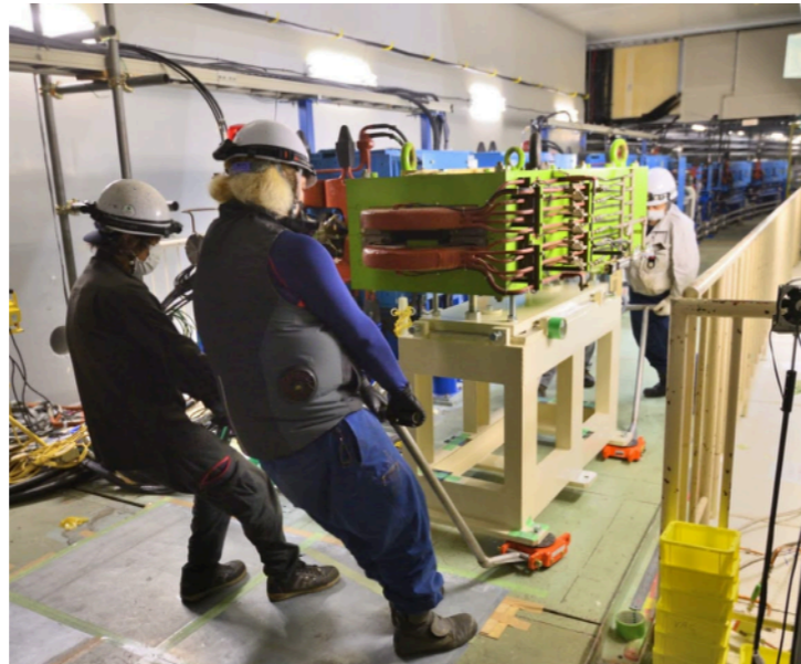
Transfer and installation of dipole magnet
