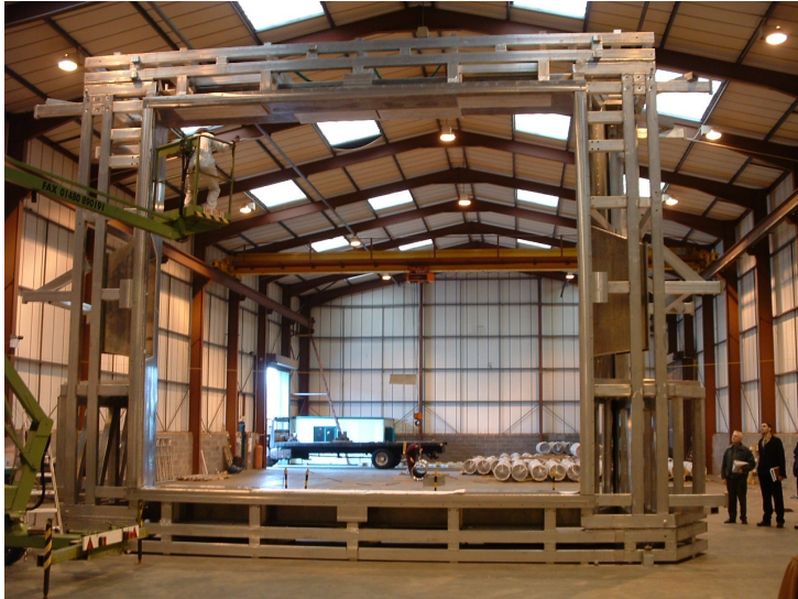
RICH2 super structure
