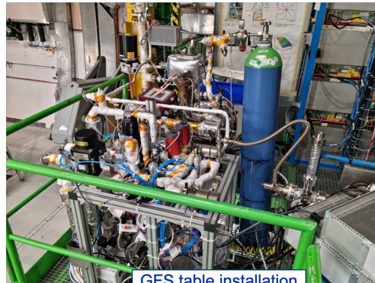
GFS table installation
