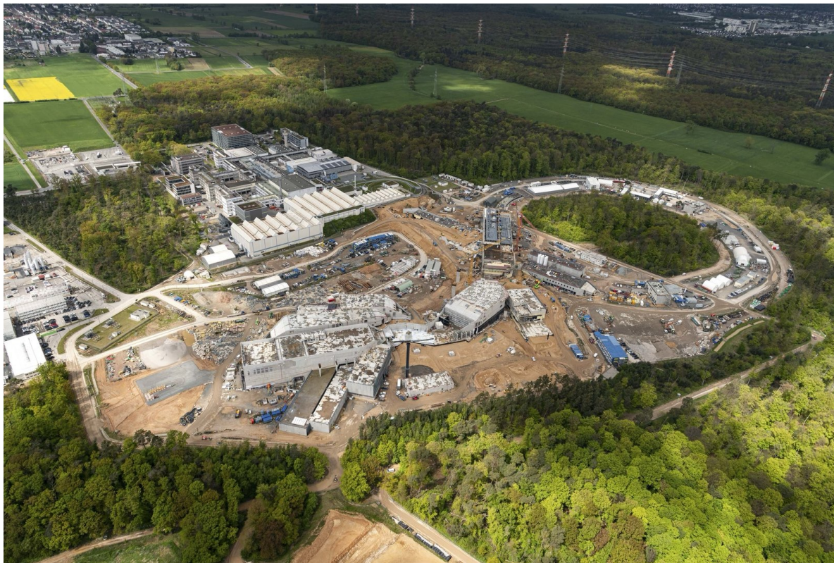
Shell construction of accelerator tunnel finished
