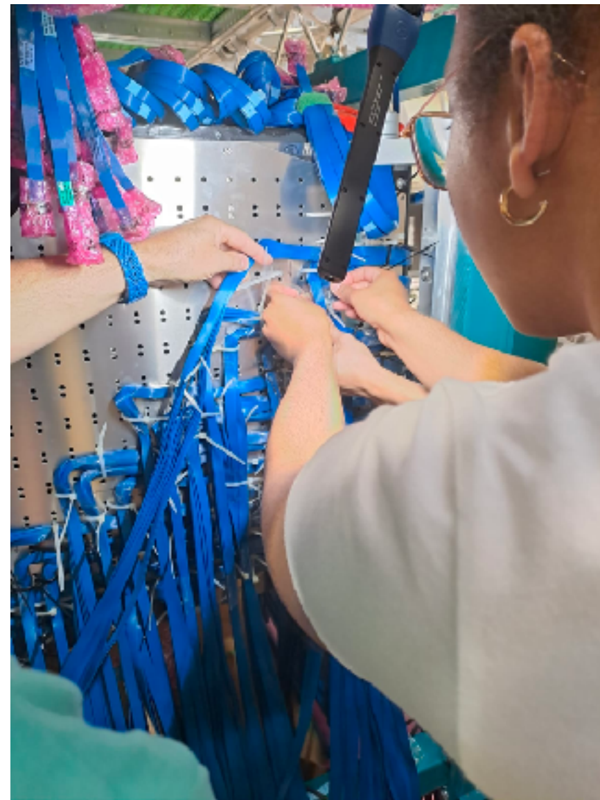
Lena working on arranging the cables.
