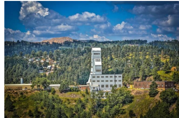
Surface infrastructure (Ross Shaft) of the mine in the Black Hills
