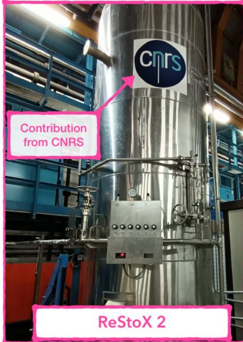
New fast recovery system to handle our larger xenon inventory
