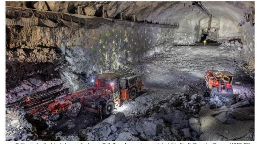
Drilling holes for blast charges for bench C (left) and removing muck (right) in North Detector Cavern (4850-33)
