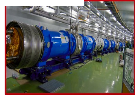
J-PARC facility: neutrino beam
