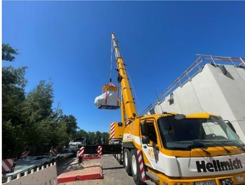
Using a mobile crane to unload a 60-tonne multiplet from a lorry and carefully guiding it into the L0317A hall (Low Energy Cave)
