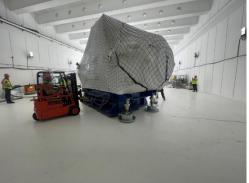
Positioning the multiplet in the L0317A hall using air cushions and a forklift for smooth and accurate placement
