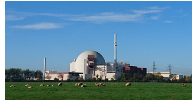
Nuclear power plant (Brokdorf, KBR)
