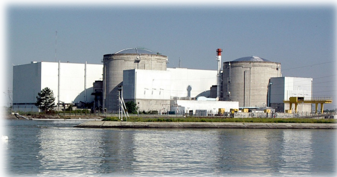
Nuclear plants (dismantling)
