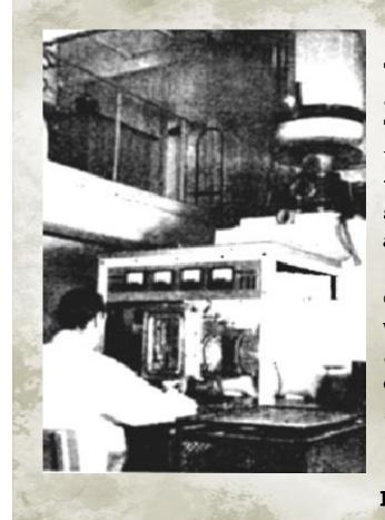
NBI isotope The separator in 1951. The elements are the high voltage terminal and ion source (top), the analyzing magnet (behind), and the dispersion chamber with the collector slit used in the experiment (in front).
