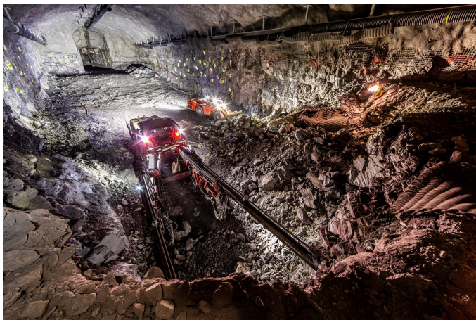
North detector cavern
