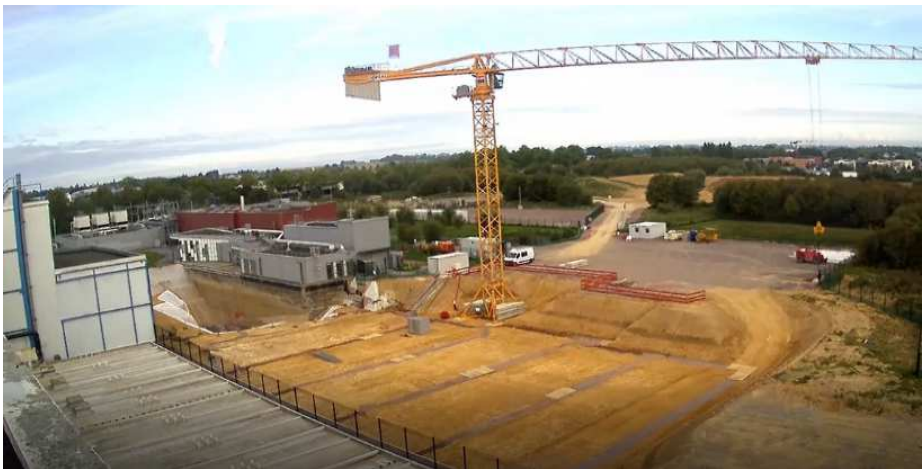
September 2023: Building construction preparation
