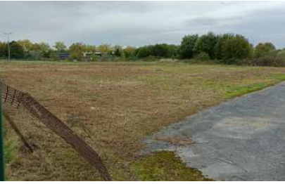
October 2022: Site preparation
