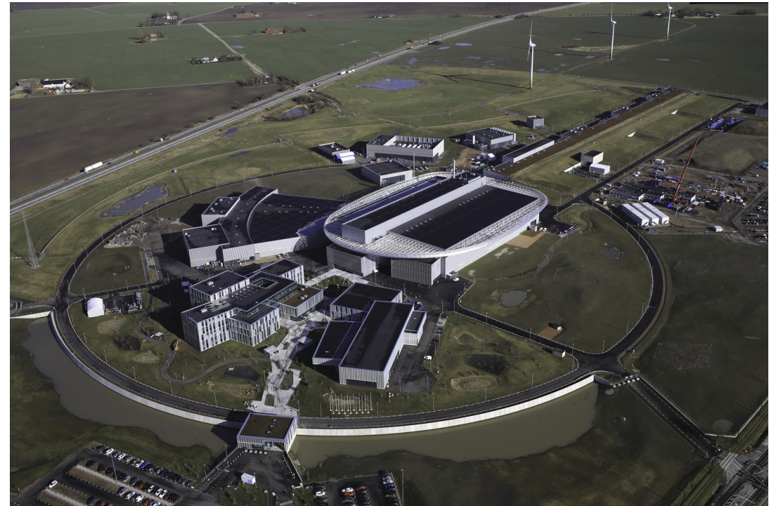
Aerial view of the ESS site February 2022 (Image from Perry Nordeng)
