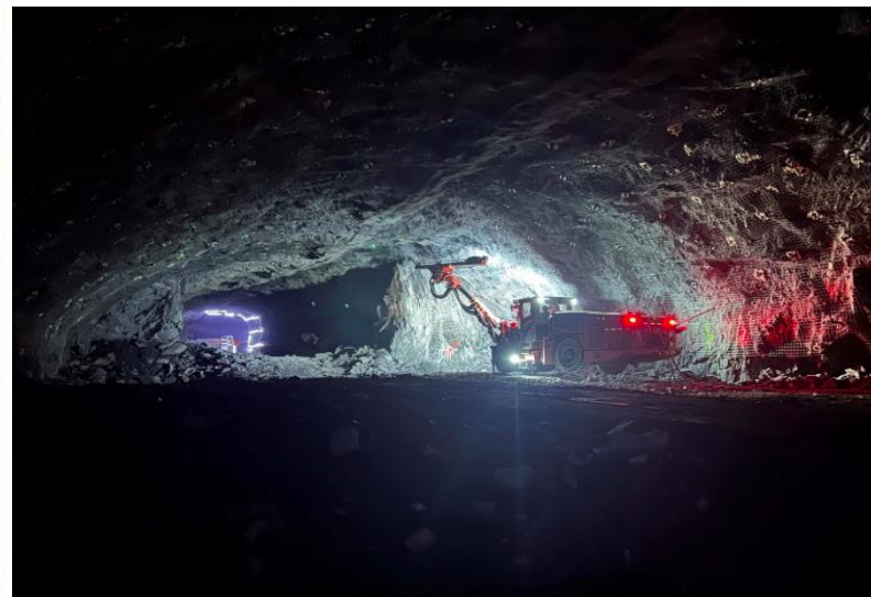
Drilling holes for blast charges in Central Utility Cavern (4850-36)
