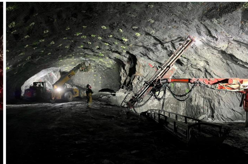
Installing CT Rock Bolts in Central Utility Cavern (4850-36)
