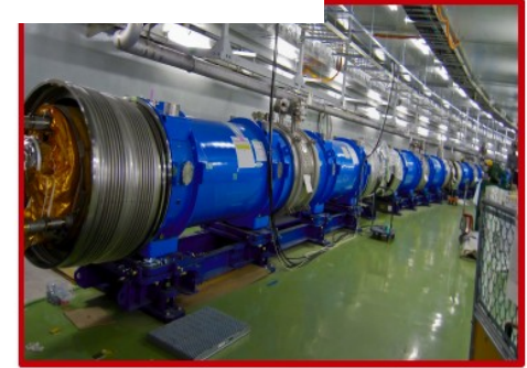
J-PARC facility: neutrino beam
